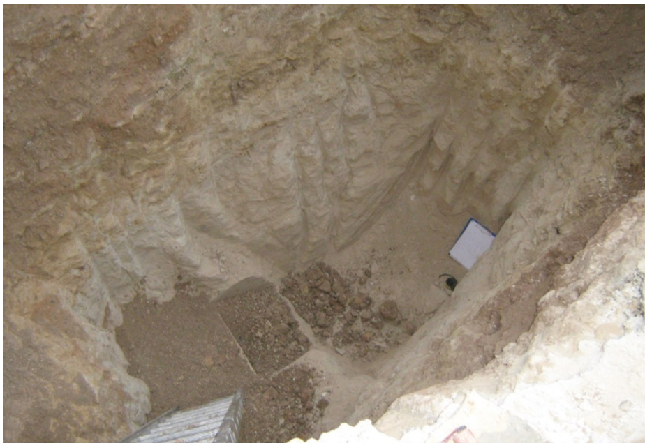
Figure 2 - Trial pit excavated below the West front, October 2012
